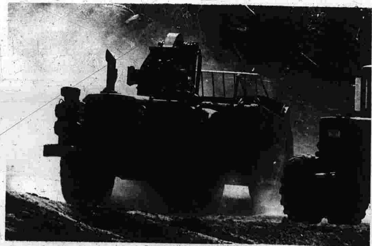
Carrying 25 Yards of Earth
